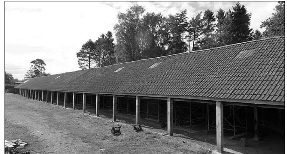
Dawes Twine Works undergoing renovation
